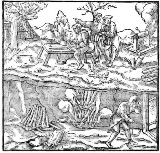
A-KINDLED LOGS. B-STICKS SHAVED DOWN FAN-SHAPED. C-TUNNEL.
